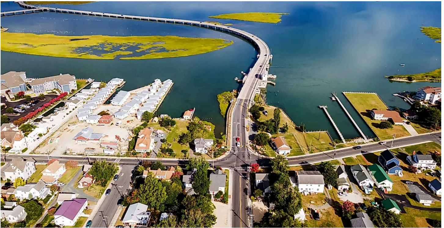
The Chincoteague Bridge across Chincoteague Bay in Virginia.
